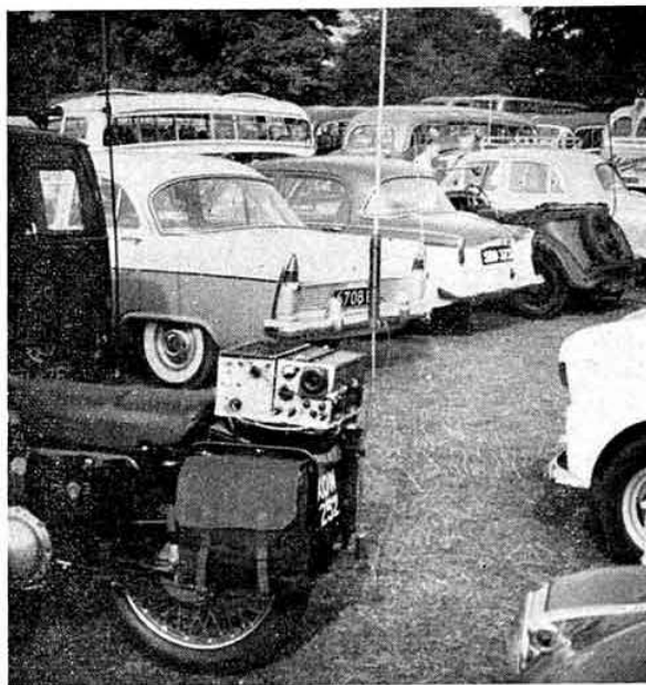
G3IVP/M won the prize for the most interesting rig at the Woburn Abbey National Mobile Rally on September 13, 1959, with his Top Band s.s.b. mobile transceiver, shown here mounted on the back of his motorcycle XOW252.
